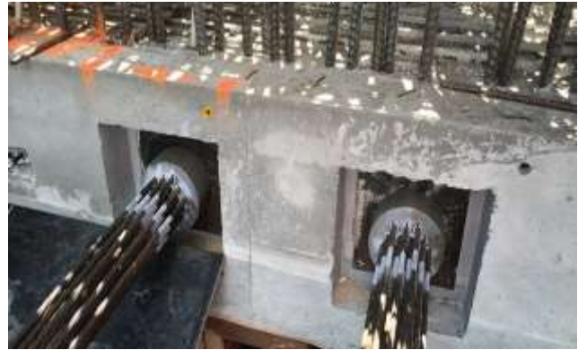
Figure 2-11 Multi-strands application ( http://www.tensionedconcrete.com.au/post-tensioning-services/ , 2021)
