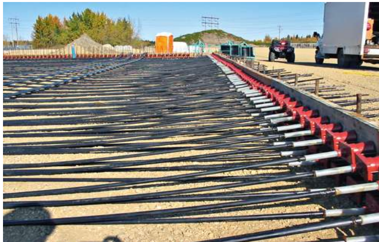
Figure 2-12 Mono-strands system application ( https://www.dywidag-systems.com/projects/2009-info-17/dsi-monostrand-system-prevents-loss-of-material/ , 2021)
