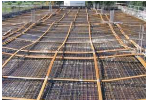
Figure 2-3 Post-tension concrete slab before concrete casting ( https://theconstructor.org/structural-engg/pre-engineered-building/ , 2021)
