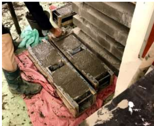
Figure 4-16 Standard concrete cube molds (left) and concrete standard cubes casting and compaction (right) (top) and concrete standard cubes leveling (bottom)
