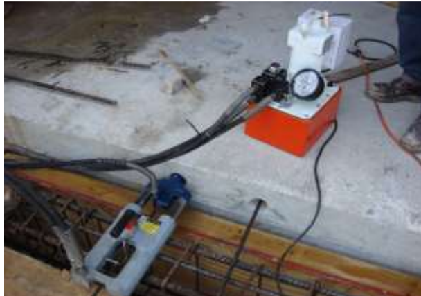
Figure 2-2 Hydraulic jack and prestressing machine (PTE SYSTEMS INT'L. LLC).
