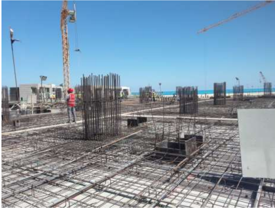
Figure 1-1 New Almain towers post-tension bonded slab under construction
