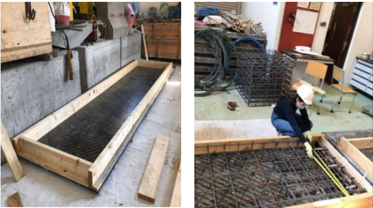
Figure 4-2 Slab specimen formwork (left) and checking the internal dimensions of the slab specimen formwork (right)
