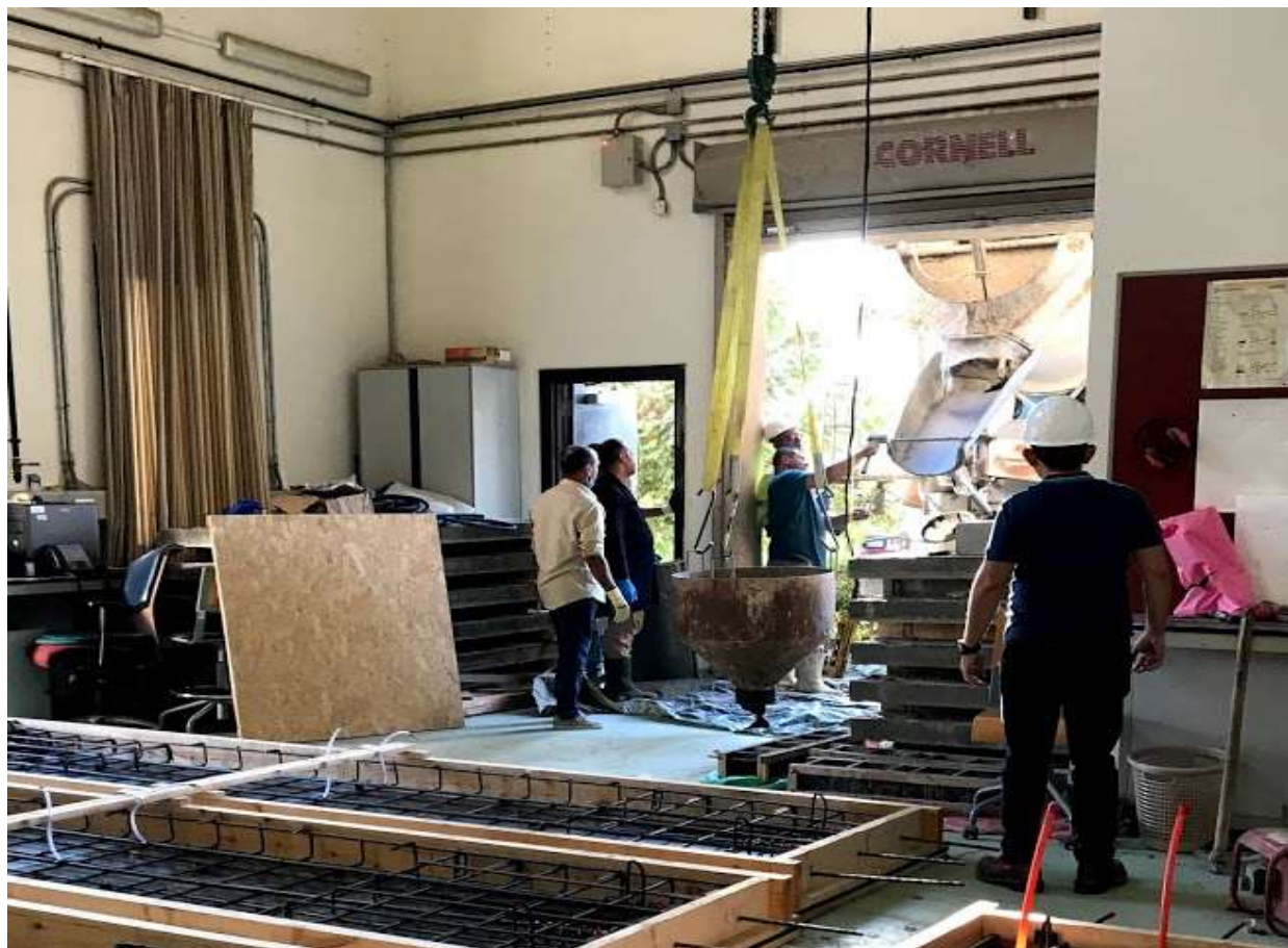
Figure 4-14 Rotating drum delivering concrete to the AUC lab
