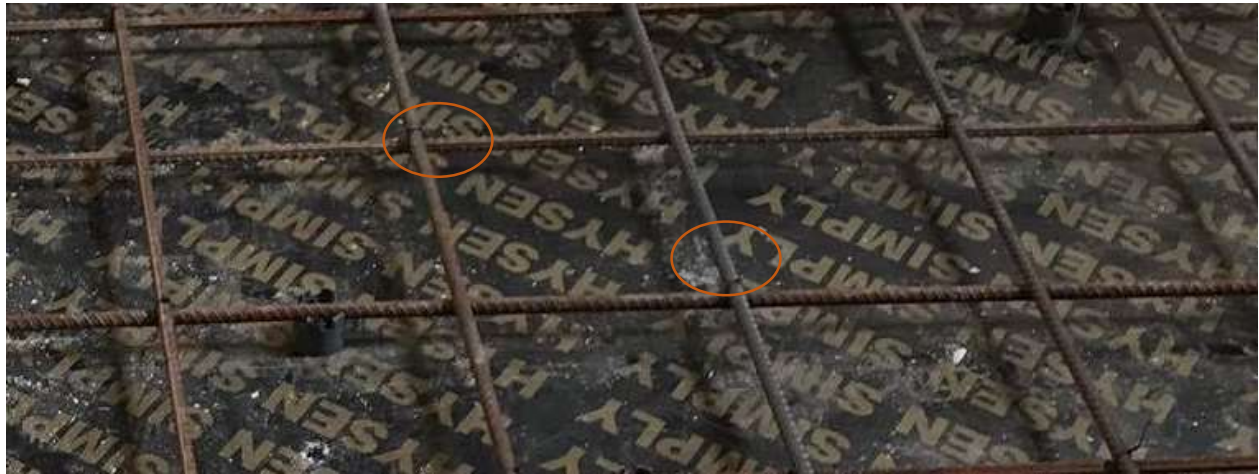
Figure 4-4 Wires connecting the steel bars in the slab specimen
