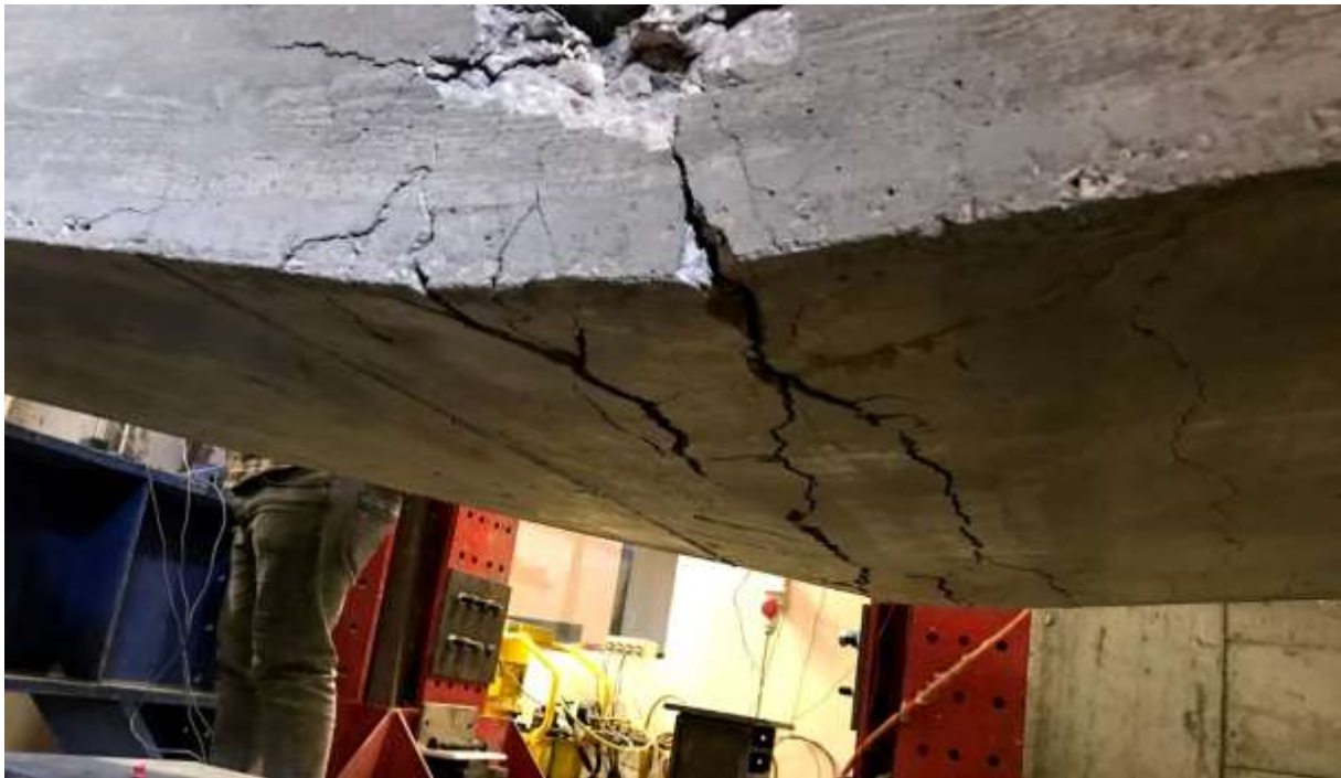
Figure 5-6 Major cracks at the bottom surface of the concrete slab at failure located at mid-span
