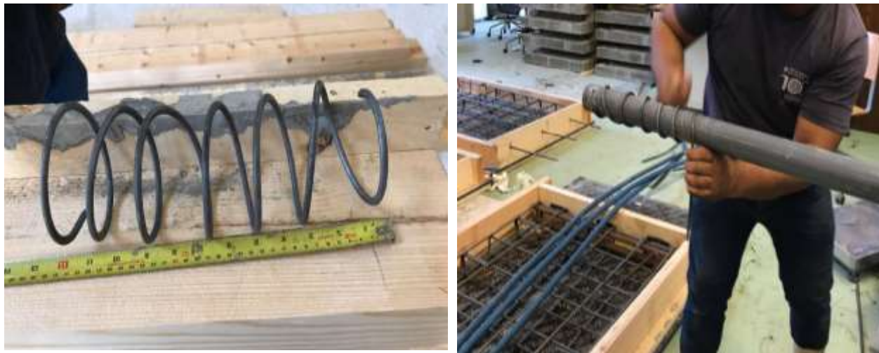
Figure 4-5 Spiral Stirrups Before Erection showing the total length of the stirrup (left) and spiral stirrups formed in the lab manually (right)
