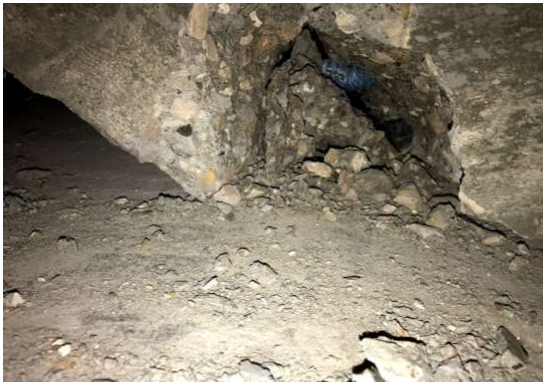
Figure 5-15 BS2 completely fallen down to the ground after a few seconds from stopping the test (top) and one of the tendons in BS2 was detected unbroken after failure (bottom)
